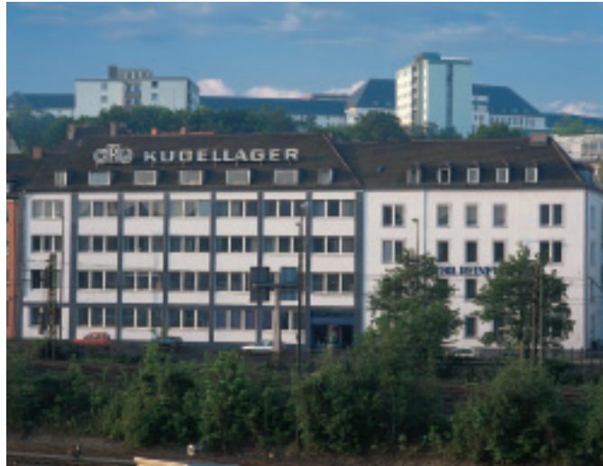
Administration and production facilities in Würzburg
